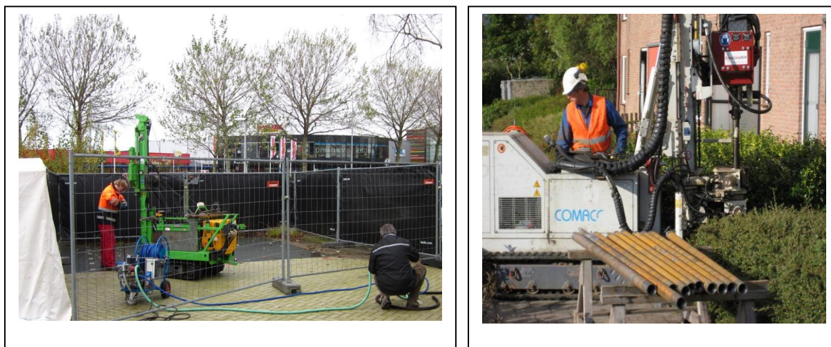
Figure 2. Photos of direct injection of carbon source to stimulate biological degradation.
