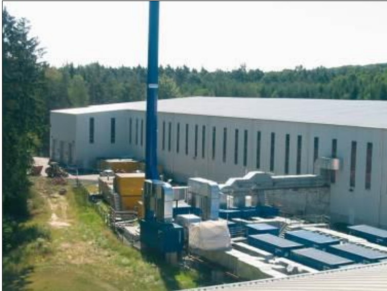
Fig. 5: Remediation of TRI-Halde
